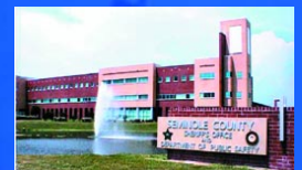
Public Safety 150 Bush Blvd, Sanford, FL
